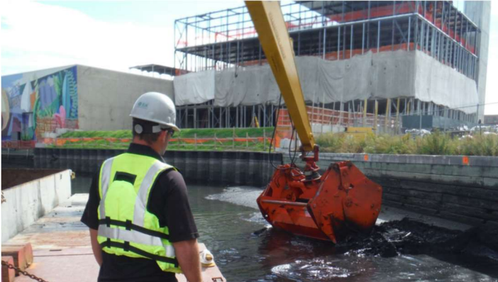
Excavator removing sediment from Gowanus Canal 4 th Street turning basin in 2018
