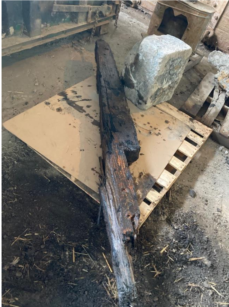
Photograph 8 – Notched timber, front view.
