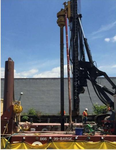
*Auger mixing cement into contaminated native sediment during pilot ISS in 7<sup>th</sup> Street Turning Basin (conducted in 2015)*
