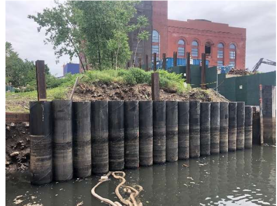
Figure 1: Pipe Pile Bulkhead at the 1 st Street Turning Basin
