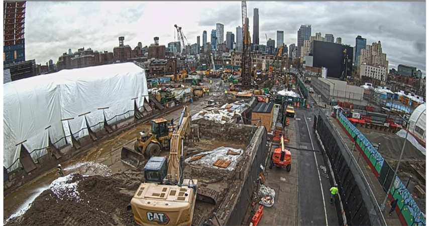
8-million-gallon tank site during perimeter wall construction
